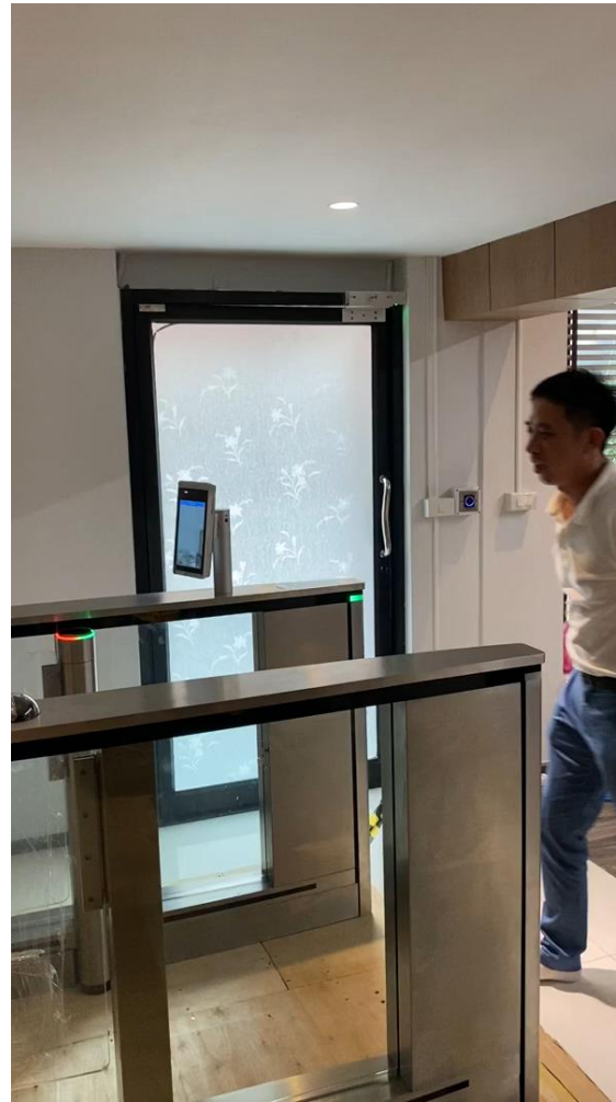
Demo Gate Barrier with Face Recg
